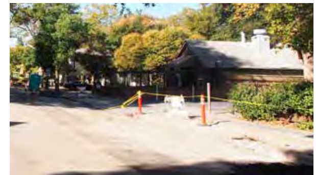
Ongoing Stormwater & Sewer Upgrade (Third Street)
