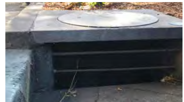
Characteristic Existing Stormwater Inlet
