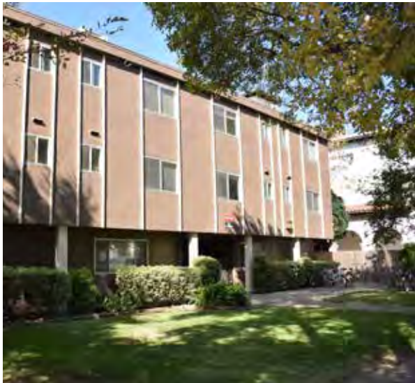
Frontages are not consistent in their quality and often do not contribute to the public realm along the street.
