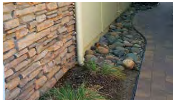
Low Impact Development Strategy - Downspout Disconnect at Sherman Townhomes to allow rainwater percolation
