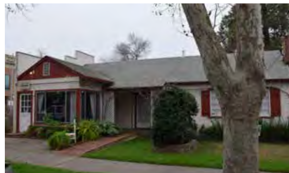
House with a shopfront addition
