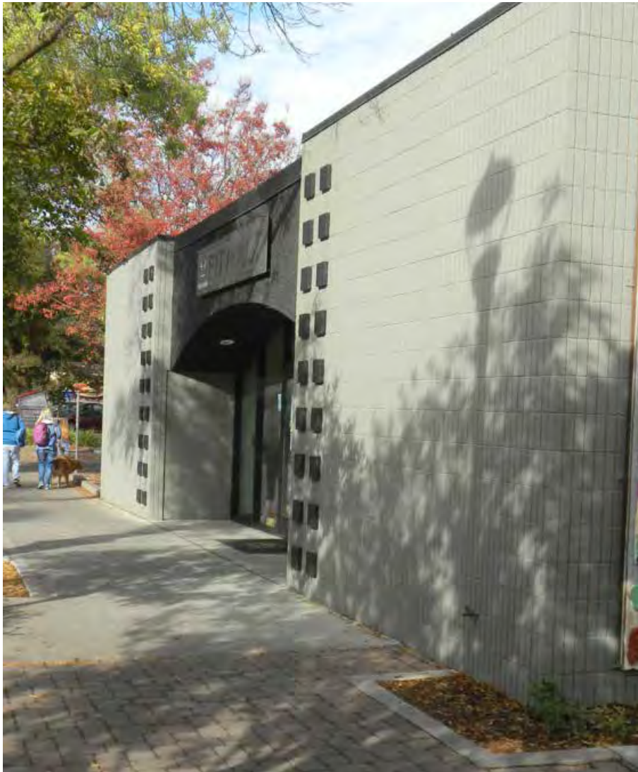
302 G Street (former Davis Enterprise newspaper plant, 1966)
