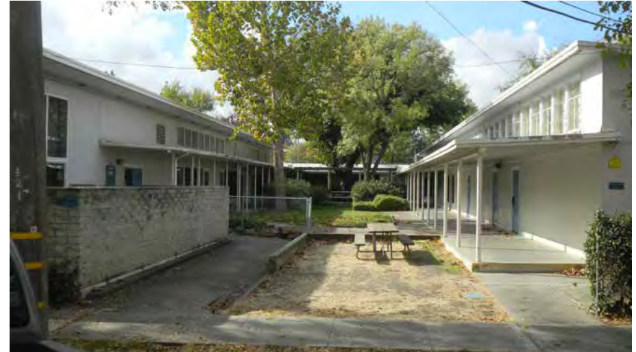
526-530 B Street (Old Emerson Jr. High School, 1949)
