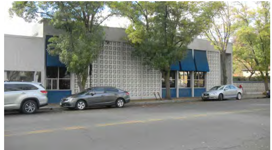
315 G Street (former United States Post Office, 1966)
