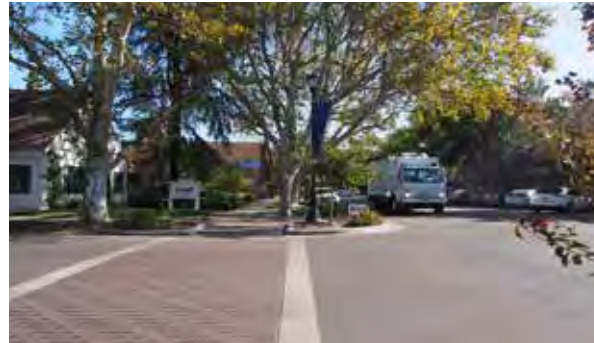
Existing Drainage Condition (Second Street)
