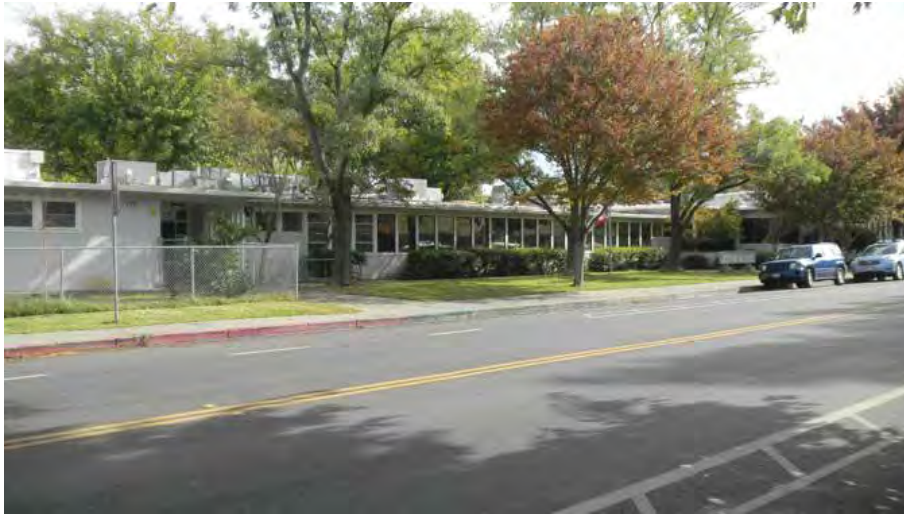
526-530 B Street (Old Emerson Jr. High School, 1949)
